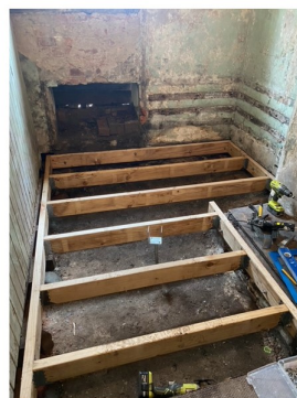
Above: Most of the below floor 'mess' cleared & new floor joists laid.
