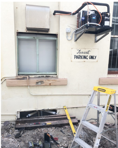
Above: work extended to the outside.
